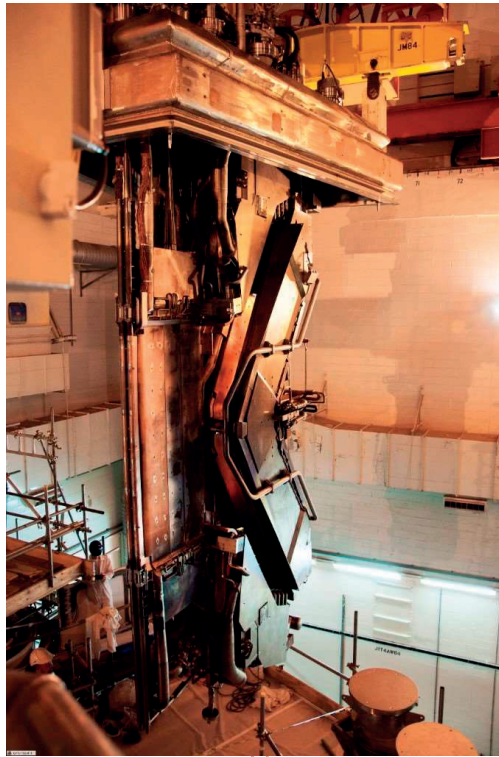
FIG. 11.57. Lifting of the JET NBI central support column.
