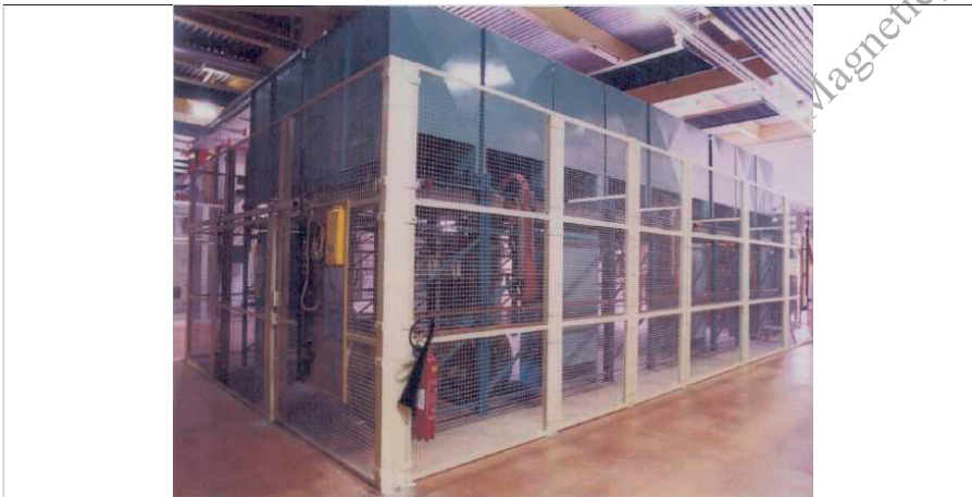
FIG. 5.33. The stainless-steel resistor bank of Tore Supra.
